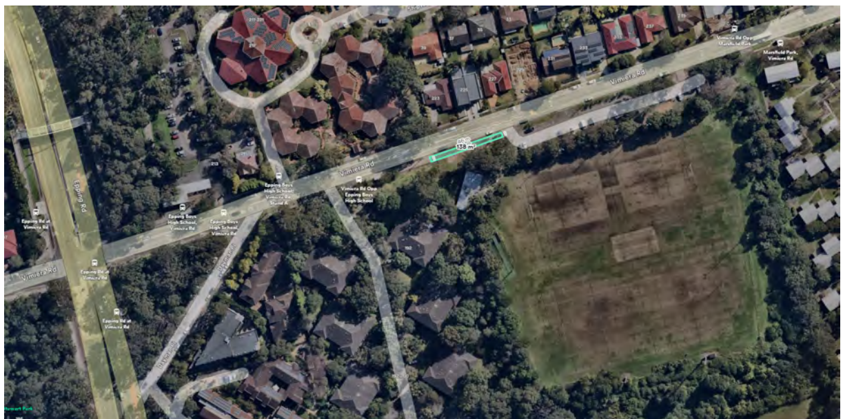
Figure 1: Vimiera Road (Epping Road - Marsfield Park)
