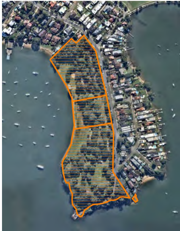
Image 2: Site Overview - Putney Park.
