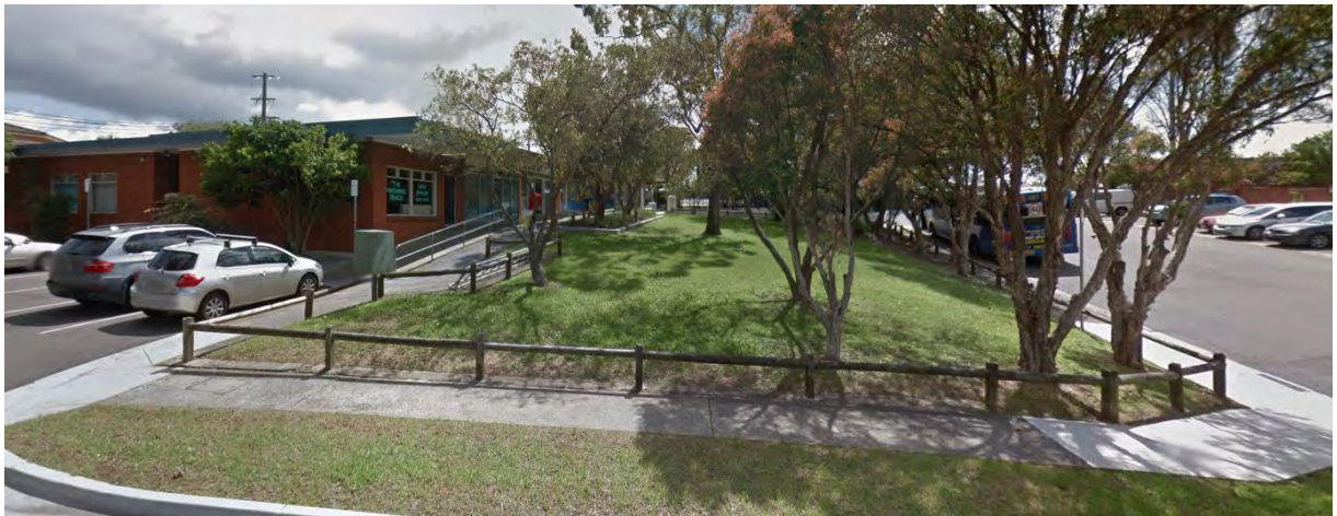
Figure 3 – Corner of Sager Place and Moncrieff Drive prior to signage and power pole installation circa. 2015.
