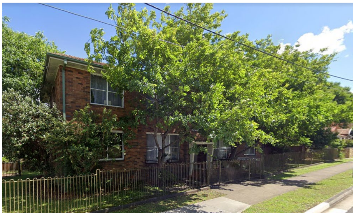
Figure 6: 17 Wattle Street - a 2 storey RFB owned by the Department of Housing. Front of building faces Anzac Ave.
