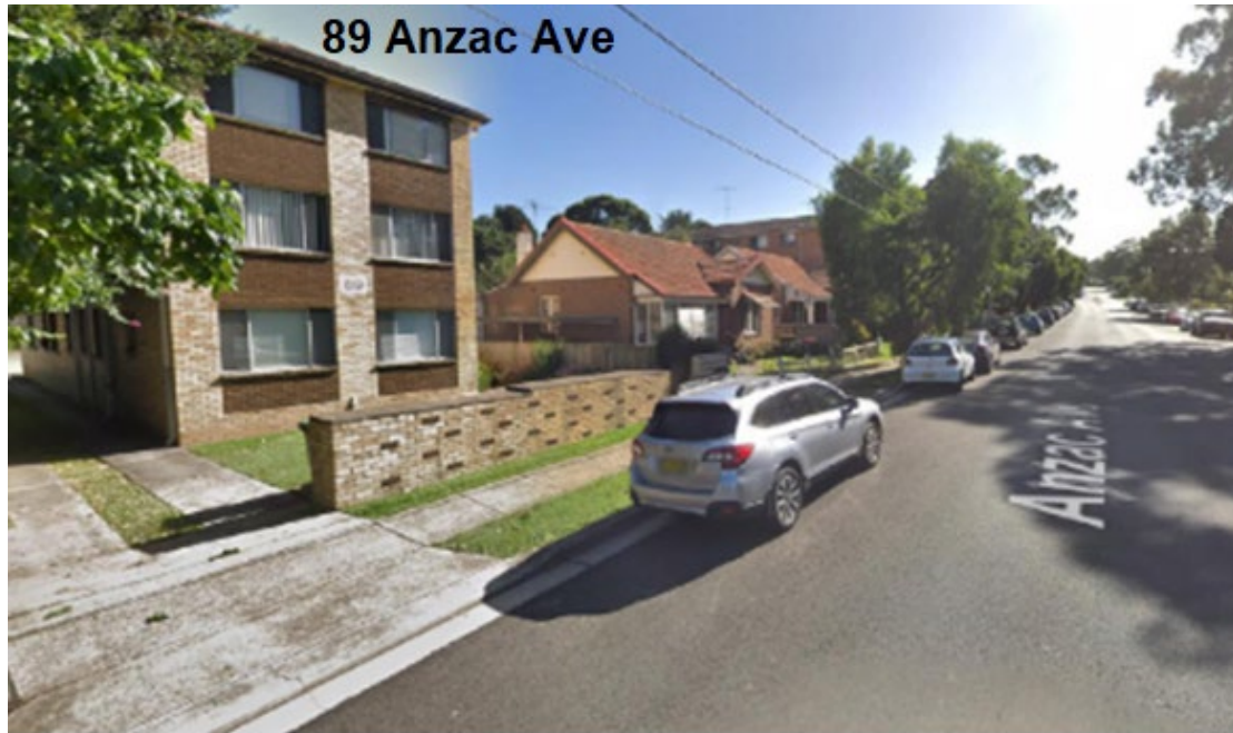
Figure 5: View looking to the north west along Anzac Ave, north east of the site. The property at 89 Anzac Avenue adjoins the rear boundary of the subject site.
