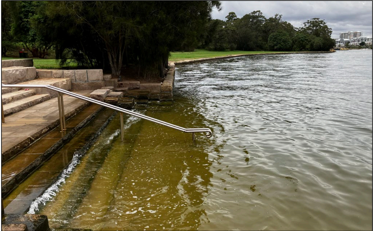
FIGURE 4: EXISTING STAIRS TO WATERWAY, LOOKING SOUTH
