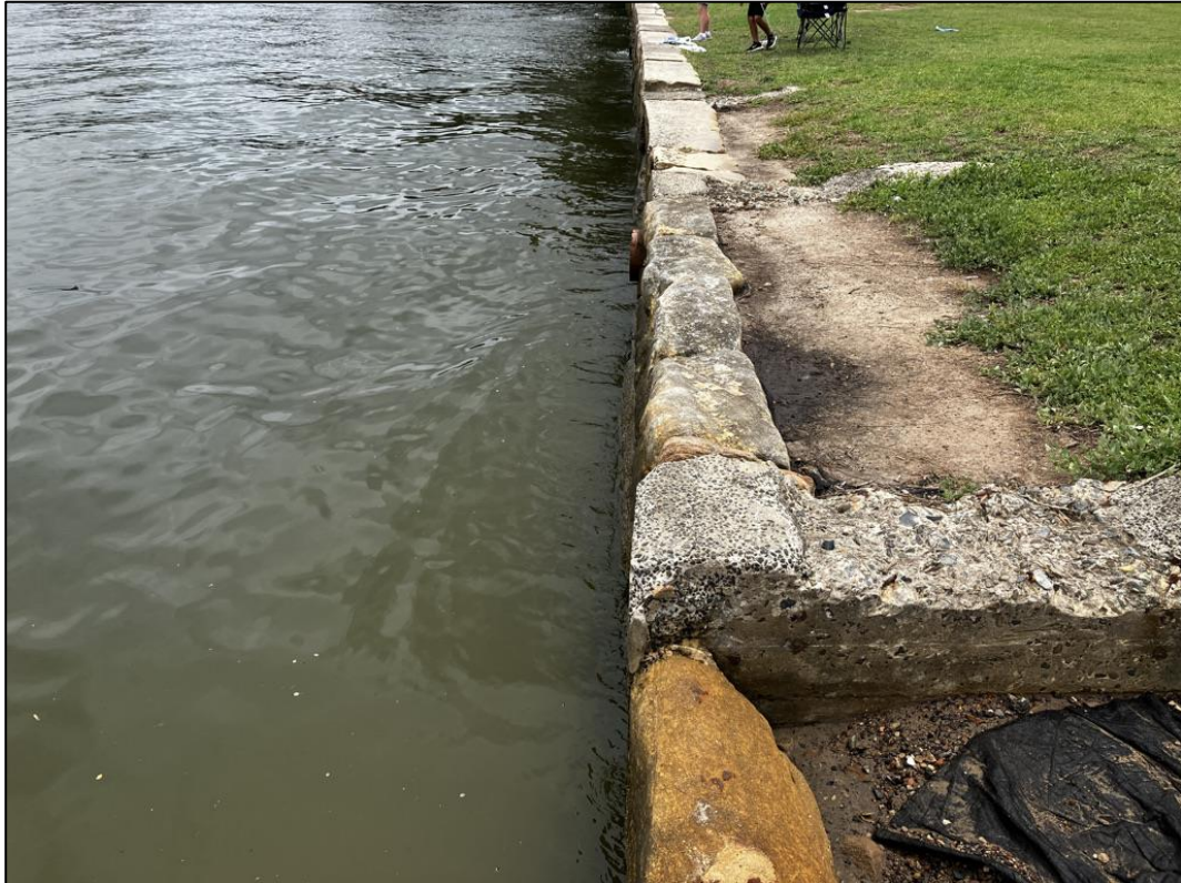
Figure 4 – View of existing sandstone sea wall along river edge.
