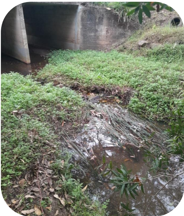
Figure 13 Shrimptons Creek at Bridge Road looking downstream (Autumn 2024)
