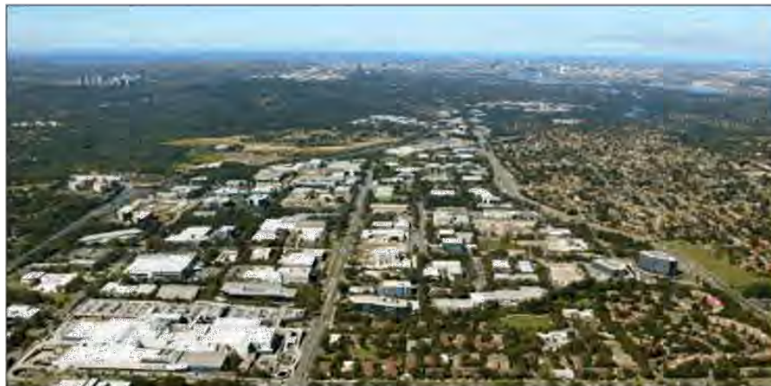
Figure 2.0.1 View east over Macquarie Park Corridor
