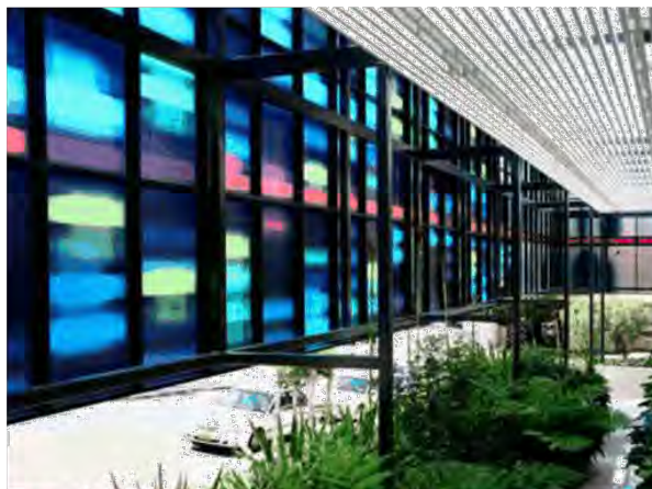
Figure 5.10.3 Police headquarters Parramatta. Here public art is incorporated into the building façade/sunscreens. The art work is based on forensic science and DNA graphs.
