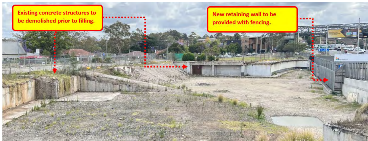
Figure 1 - photo showing works required prior to site filling.
