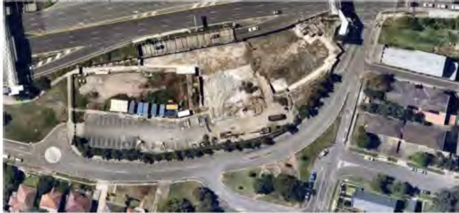
Figure 2 - Aerial photo of Ryde Central dated 4 October 2021.
