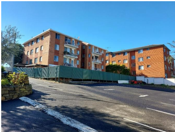
Figure 9 – Western side of 820 and rear of 822 Victoria Road
