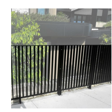
9 FRONT BOUNDARY FENCE. BLACK METAL VERTICAL BLADE FENCE. REFER TO DETAIL 3 / DA2101 - FRONT FENCE ELEVATION
