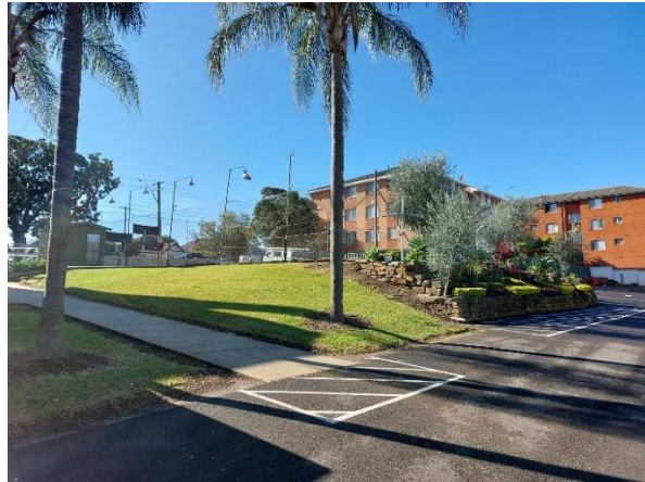
Figure 8 – View east towards the western side of 820 & rear of 822 Victoria Road
