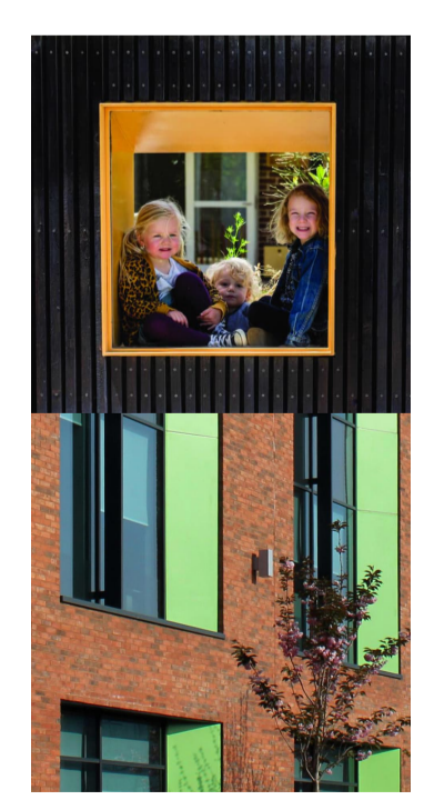
6 WINDOWS WITH COLOURED REVEALS
