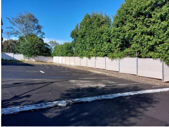
Figure 11 – View east of the rear boundary (acoustic) fence
