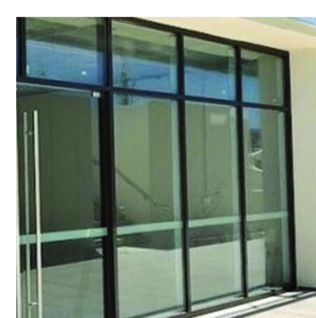
5 ALUMINIUM FRAMED GLAZED WINDOWS & DOORS - WINDOWS TO INCORPORATE OPENABLE PANELS - FRAME COLOUR: CHARCOAL
