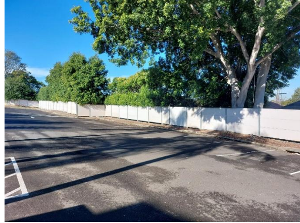
Figure 12 – Long view east of rear boundary (acoustic) fence
