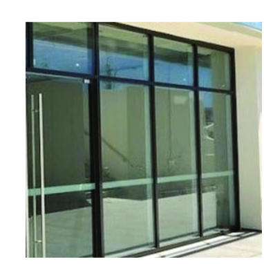
5 ALUMINIUM FRAMED GLAZED WINDOWS & DOORS - WINDOWS TO INCORPORATE OPENABLE PANELS - FRAME COLOUR: CHARCOAL ACOUSTIC MIN. REQUIREMENT (REFER TO ACOUSTIC REPORT) - MIN. 10mm THICK EXTERNAL GLAZING TO CLASSROOMS 4 & 5 SECTION J - BUILDING FABRIC REQUIREMENTS ALL GLAZING - SYSTEM MAX U-VALUE = 4.30 ALL GLAZING - SYSTEM MAX SHGC = 0.45
