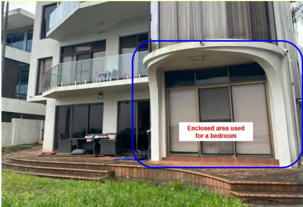
Figure 11 The existing dwelling showing the "Outdoor Covered Area", which is internalised within the dwelling and currently used as bedroom.
