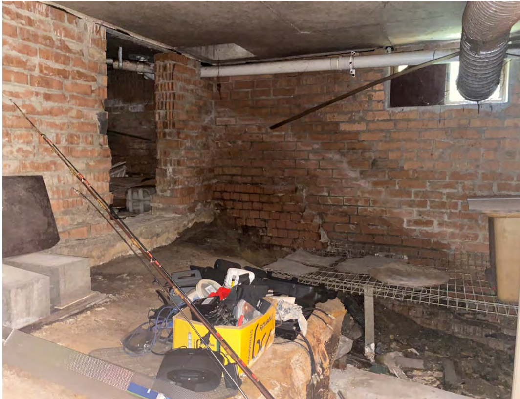
Figure 13 The 'existing sub-floor' area looking in a north eastern direction.
