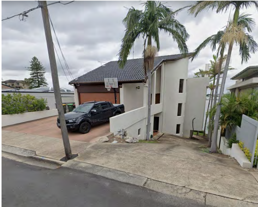
Figure 3 Southern elevation of the existing dwelling as viewed from Shackel Avenue.
