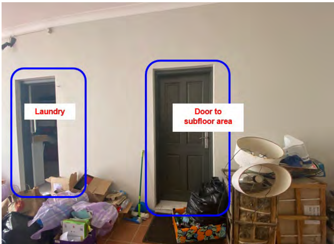
Figure 14 The laundry and bathroom at the lower ground floor level.
