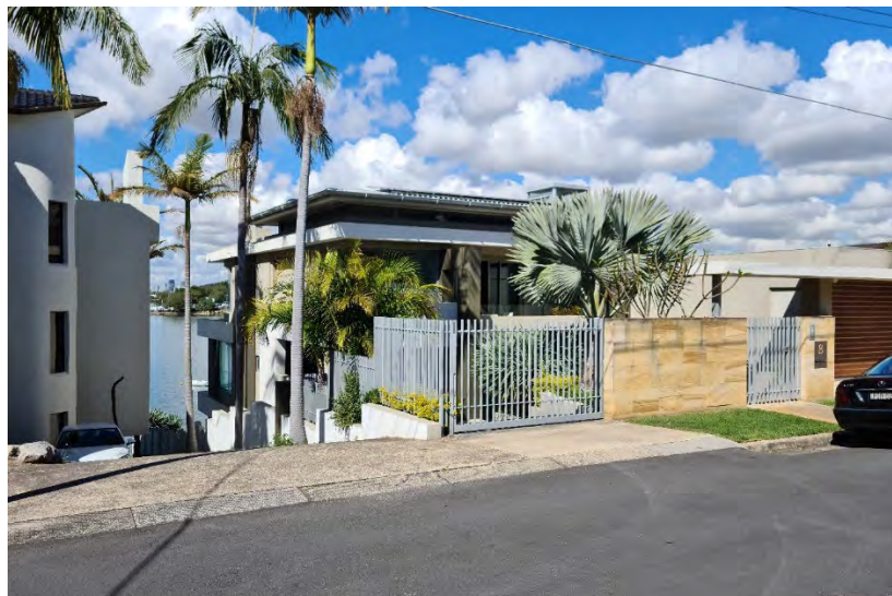
Figure 4 Adjoining dwelling situated at 8 Shackel Avenue.
