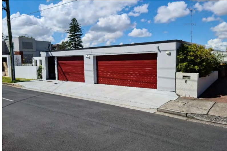
Figure 5 Adjoining property to the east, No. 4 Shackel Avenue.
