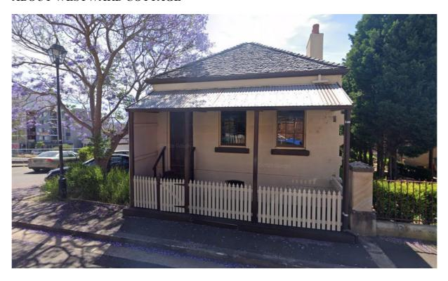
Westward Cottage is a two-storey modest Victorian workers' cottage of dressed sandstone and brick. The building was originally constructed between 1844 and 1850 and has undergone various modifications and additions.
