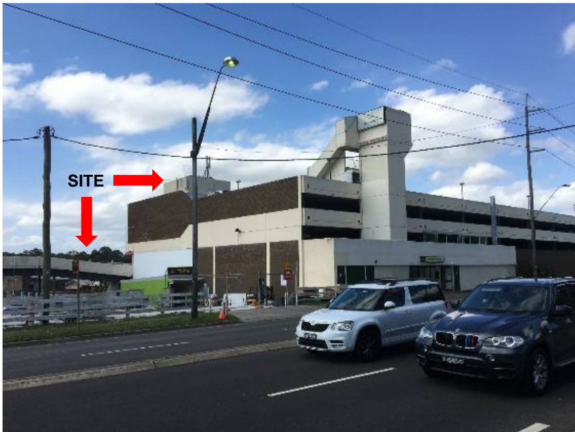
Figure 7: Looking north-east from Rutledge Street to site
